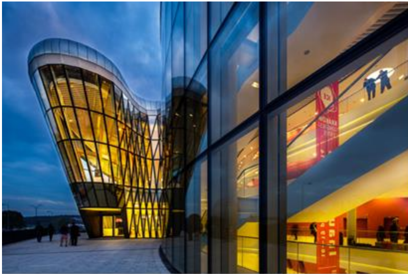
PHOTO: Silicones Secure Complex Façade of Landmark ICE Krakow Conference and Congress Center in Poland
